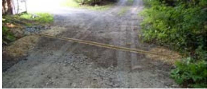
This open-top culvert at Maidstone Lake diverts water from the road to a rock apron (left), to infiltrate the ground.
