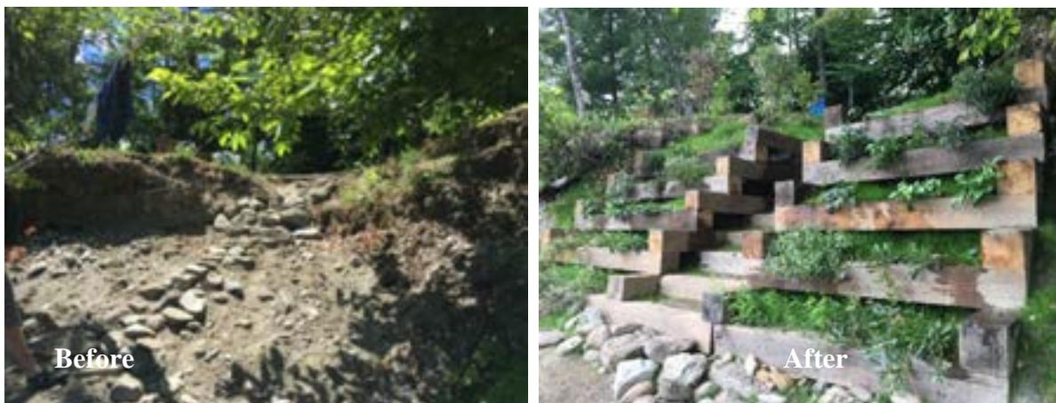
A Live Crib Wall was built to stabilize this eroding shore along Waterbury Reservoir State Park. Live Crib Walls are built from natural materials, like these untreated hemlock timbers and native plants.
