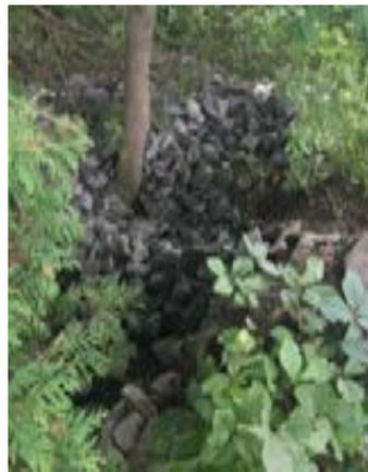
Stone check dams slow runoff while stabilizing drainage ditches. These rock 'U's slow and trap sediment runoff, cleaning the water before it enters the lake.
