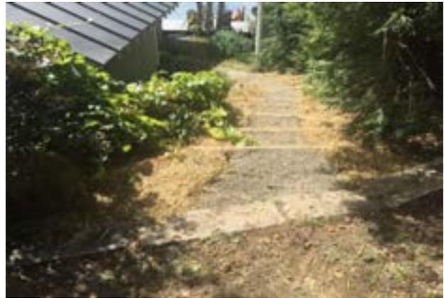
Maidstone Lake infiltration steps use crushed stone to slow and infiltrate runoff. A defined walkway also minimizes soil compaction and trampling of the shore, protecting the spongy duff layer to serve both as a nursery for seedling and to soak up stormwater.
