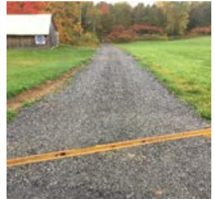
This driveway was regraded, crowned, and top coated with crushed stone. Afterwards, open-top culverts were installed to intercept and convey water to a side treatment area to protect the driveway and lake from erosive runoff.
