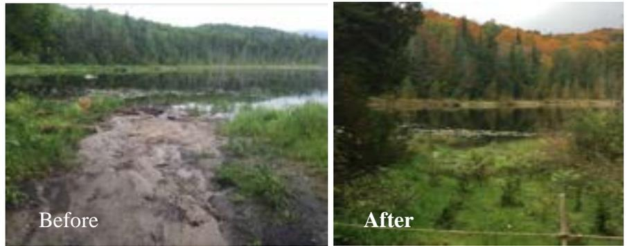
Restoring this access area called for several BMPs, starting with an upland berm or ‘speedbump’ to divert stormwater away from new plantings. Delineating a single pathway to the water will help minimize compaction, trampling, and erosion of a wider area.
