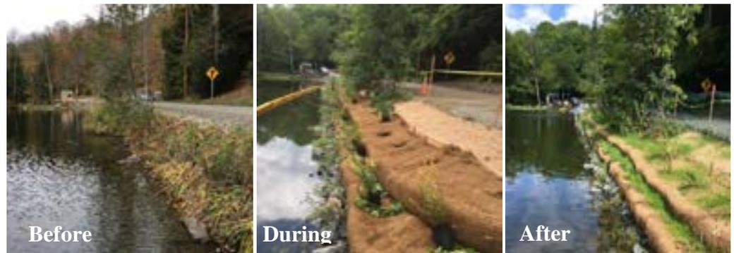
Encapsulated soil lifts reestablish a gently sloped shore, allowing native plants to root and stabilize the bank and road edge, while filtering and treating runoff before it enters the lake.
